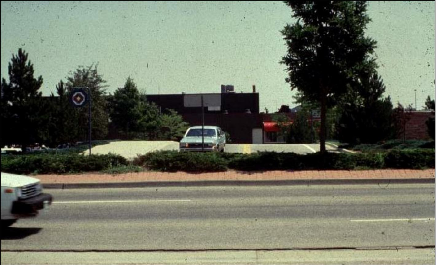
Commentary: Installation of a nontraversable median on US 36 in Boulder, Colorado, eliminated crossing and left-turn maneuvers. The landscaped median clearly communicates that the two opposing driveway are right-in/right-out only. The median landscaping provides aesthetic quality without obstructing view of the opposite side and confuse drivers into thinking the roadway on this side of the median is a 2-way street.
