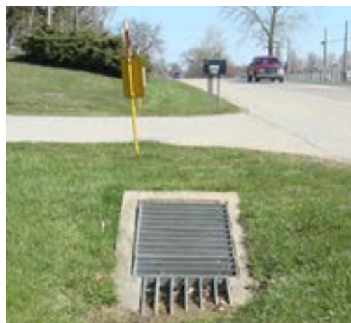
Drainage Pipe Shielding
